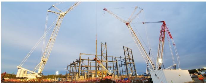
Erection of structural steel for generation building
