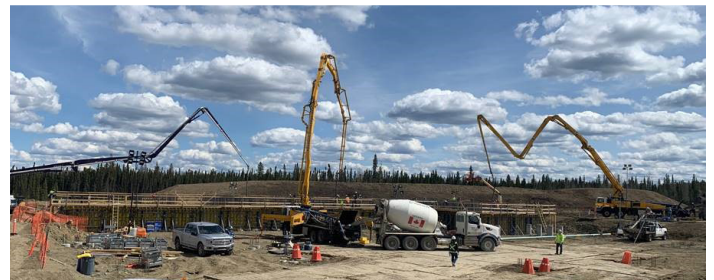
Pouring of foundation for Powerhouse
